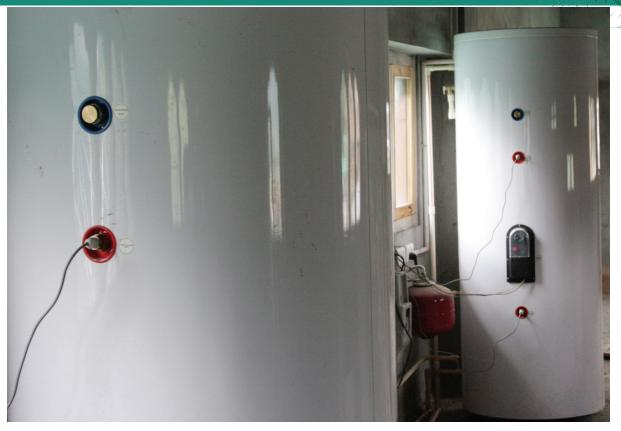
Two numbers of water storage tanks intalled with a capacity 500 litres each
