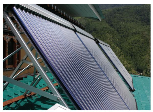
Evacuated glass tube collector installed on RSPN's roof-top
