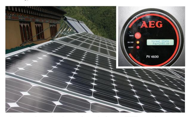
Solar power supplements the grid power in the RSPN head quarter. Inset: main DC/AC box.
