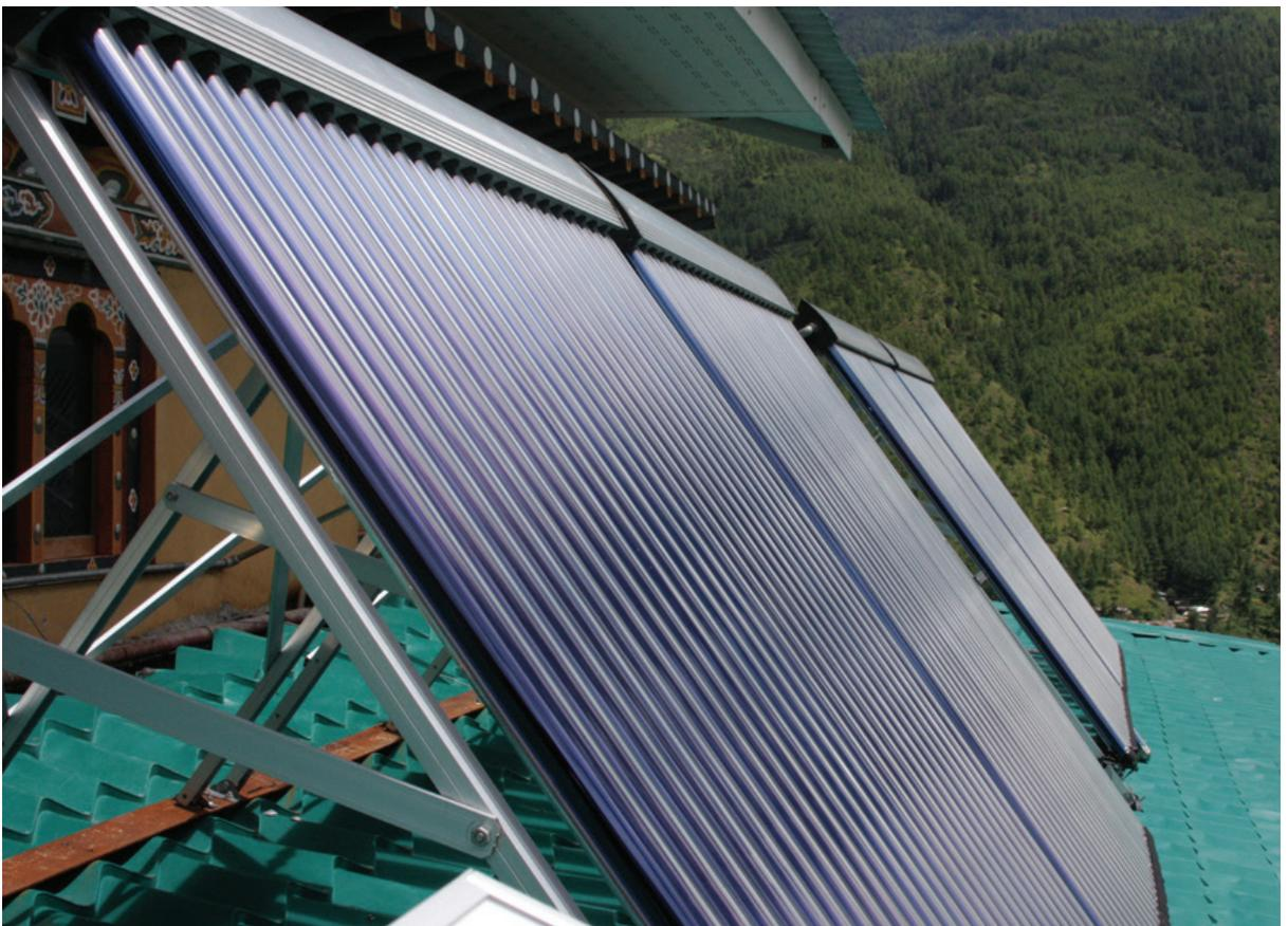
*Evacuated glass tube collector installed on RSPN's roof-top*
